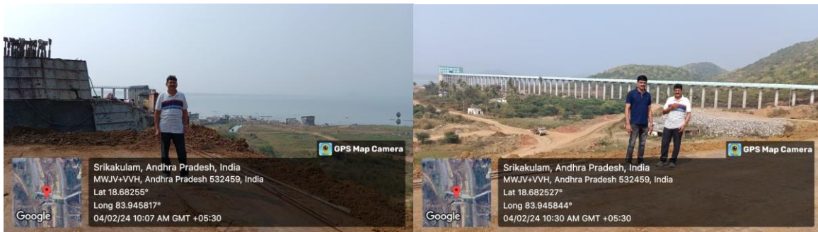
Fig. 2. Hiramandalam Reservoir outlet and Uddanam freshwater supply pipe line
