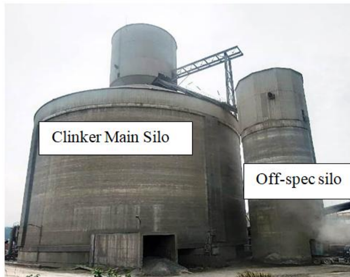
Fig. 3. An image of a main clinker silo and off – Spec silo in an existing cement plant
