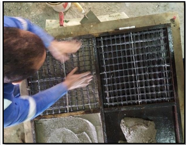
b. shows fixing the reinforcement
