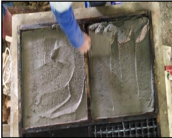
a. Shows casting of the bottom skin ferrocement layer
