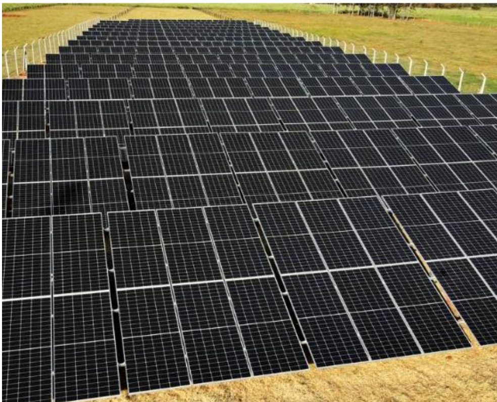
Fig. 5. Instalation of the panel
