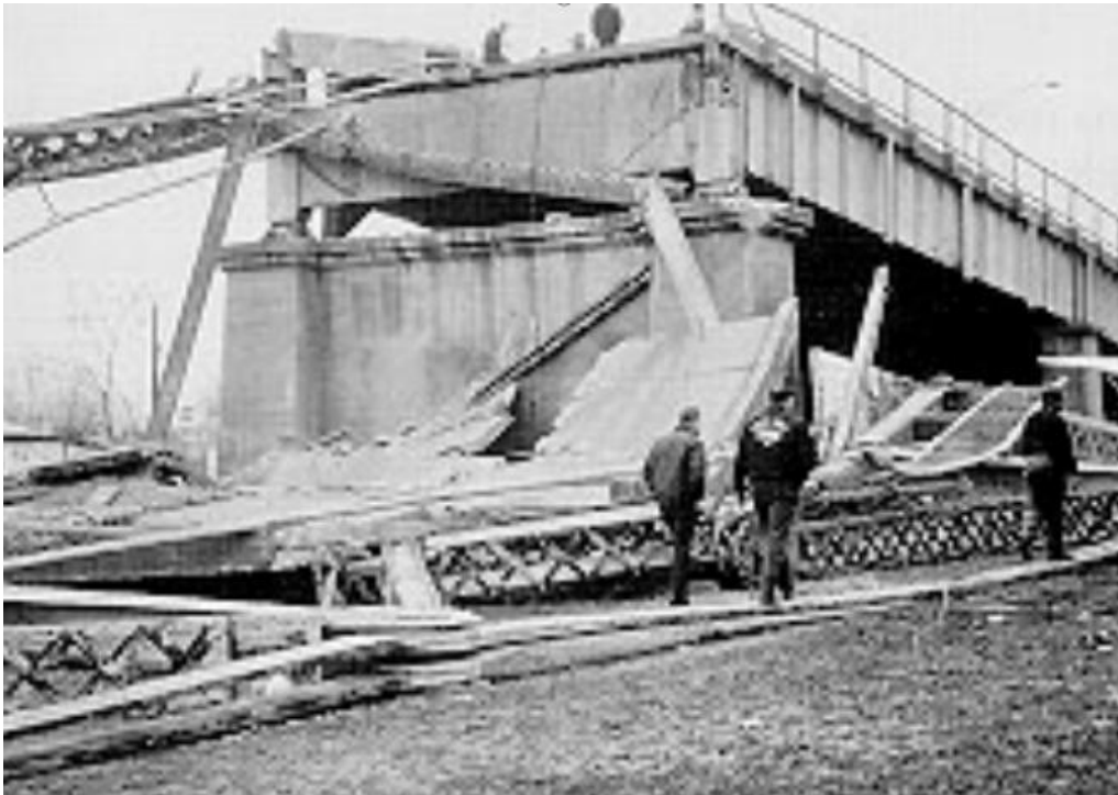
Fig. 1. Fatigue destruction accidents
